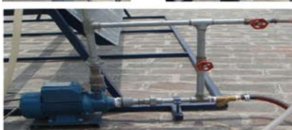
Fig. 10. Circulation System of the experimental rig.
